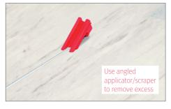
Bring the joint together and, before tightening the EasiBolts, ensure that the worktop is level along the full length of the joint.
