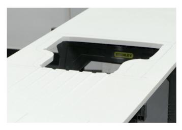
Once the adhesive has set, using a two-flute bottom bearing guide cutter, set the bearing so that it is contacting the uppermost inner face of the sink. Trim the excess material. Apply a rounded profile around the top edge of the sink. Finish the raw edge as described in the section 'Surface Finishing'.
